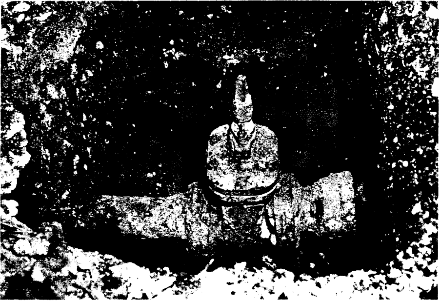
Figure 5.106a. Four-inch gate valve in water main broken by debris from brick wall (0.23 mile from ground zero at Hiroshima).
