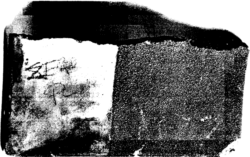
Figure 7.47. Blistered surface of roof tile; left portion of the tile was shielded by an overlapping one (0.37 mile from ground zero at Hiroshima).
