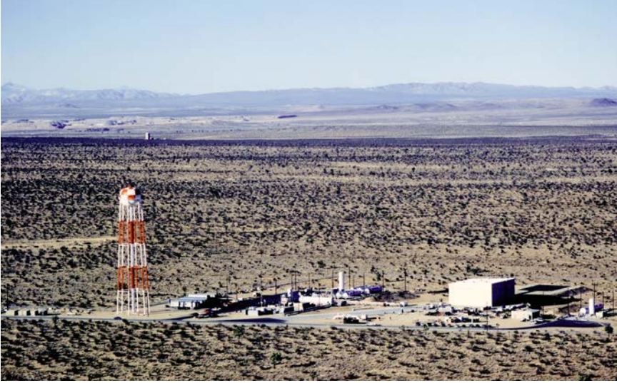
The X-33 Launch Complex that Sverdrup Corporation built on the Edwards AFB test range in anticipation of the onset of powered flight tests. (NASA)
