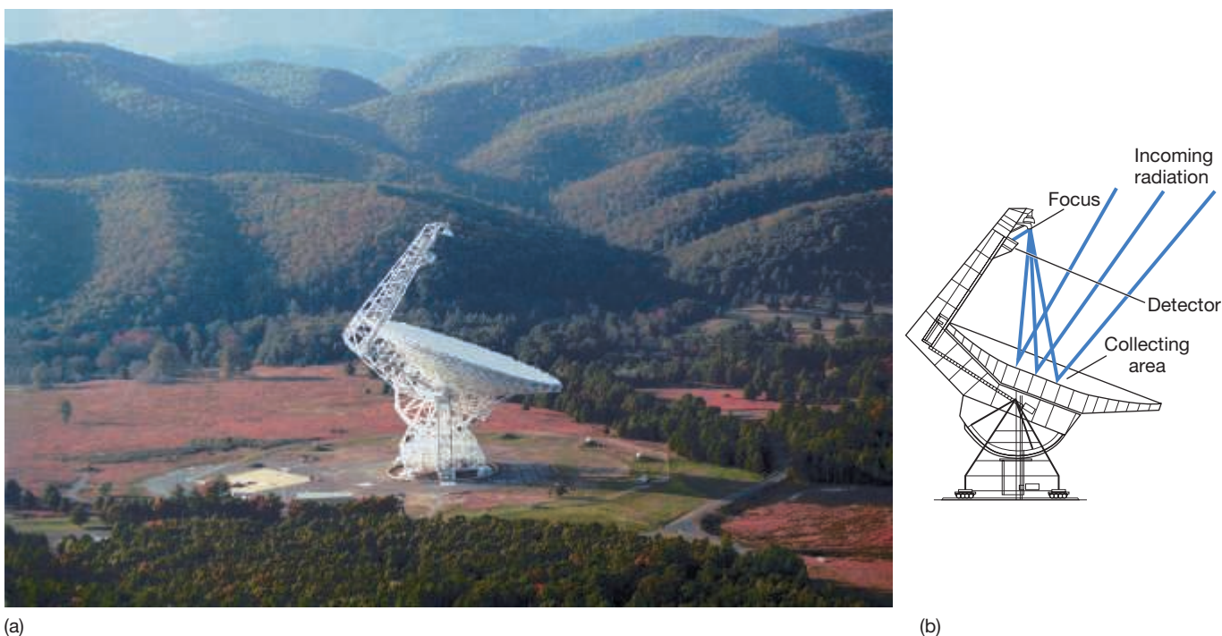
▲ FIGURE 3.16 Radio Telescope (a) The world's largest fully steerable radio telescope, the 105-m-diameter device at the National Radio Astronomy Observatory in Green Bank, West Virginia, is 150 m tall—taller than the Statue of Liberty and nearly as tall as the Washington Monument. (b) A schematic diagram shows the path taken by an incoming beam of radio radiation (colored blue). (NRAO)
