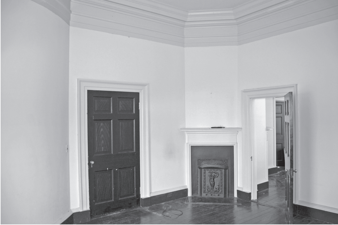
Room 203 (bedroom), looking southwest
