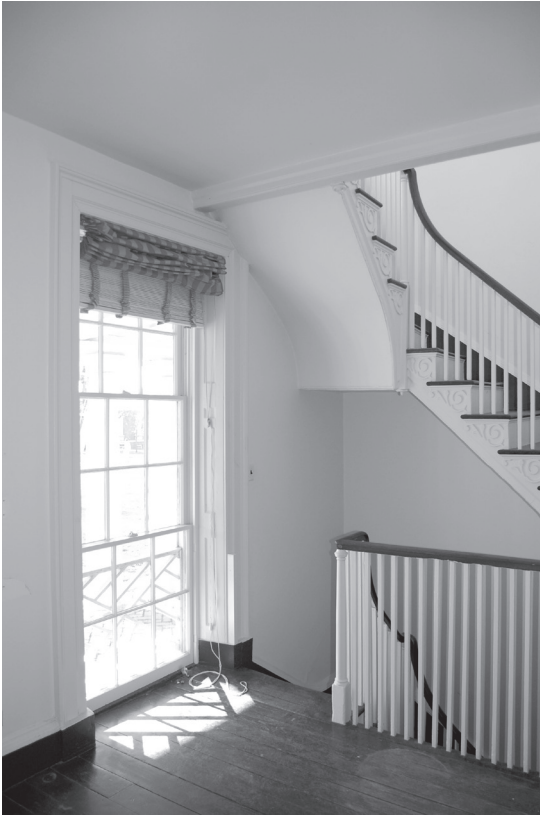
Room 104 (stair hall), looking southeast
