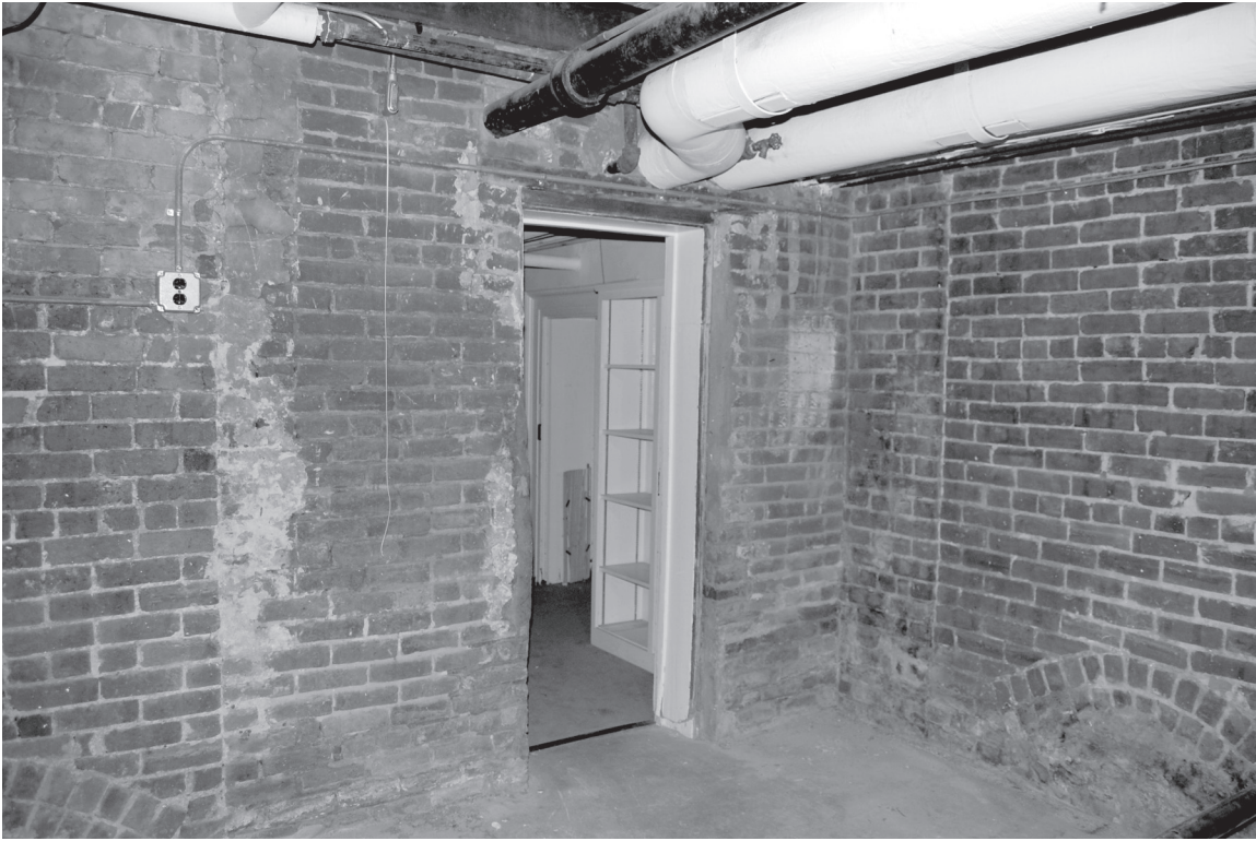
Room B11, looking northeast
