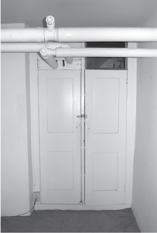
Closet in northeast corner of B07
