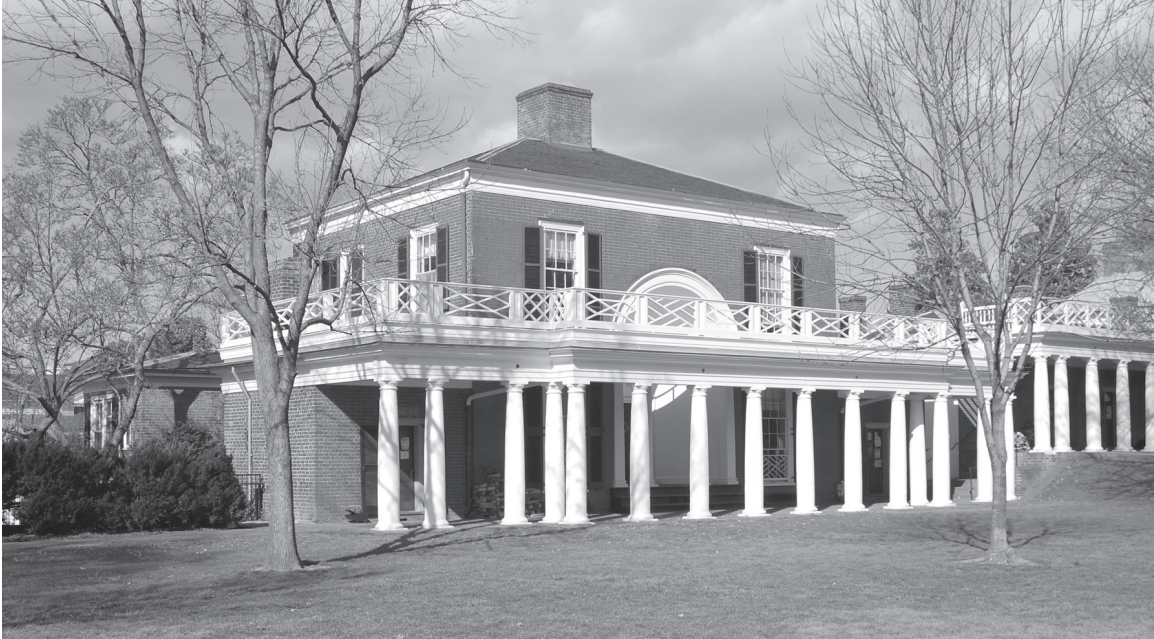
Pavilion IX from the southeast
