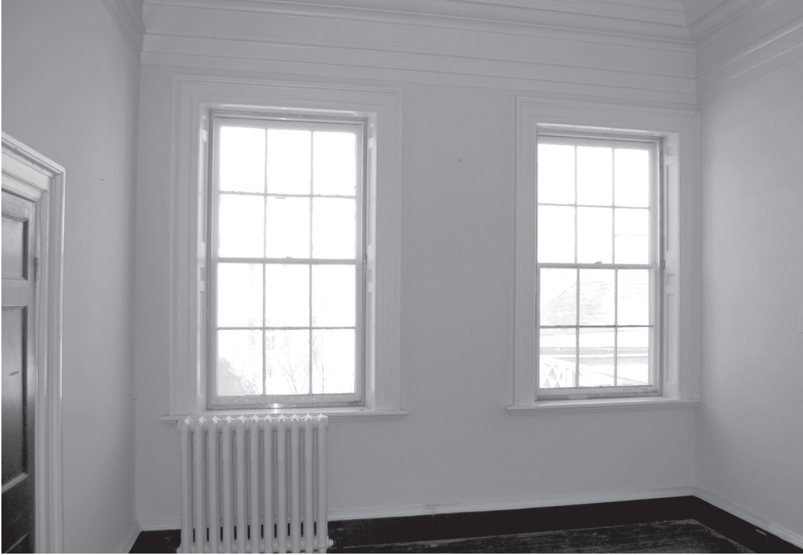
Room 204 (bedroom), looking north
