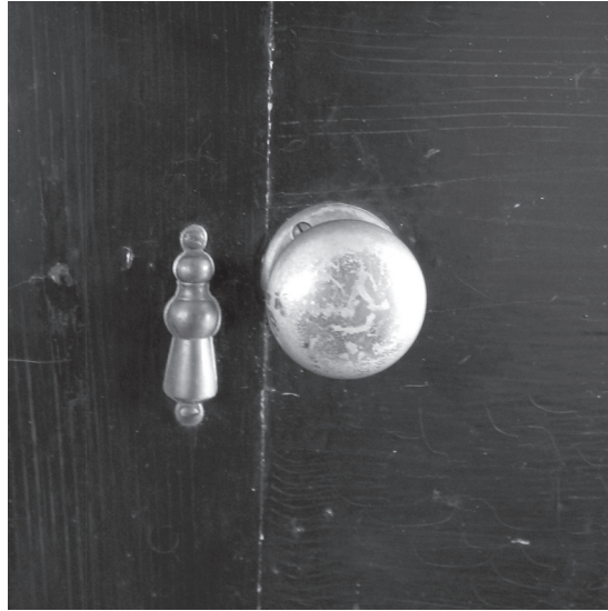
Door no. 2051 (between rooms 201 and 205), with keyhole escutcheon type A
