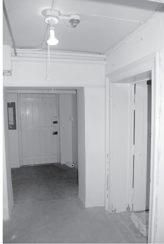
Room B03, looking west.
