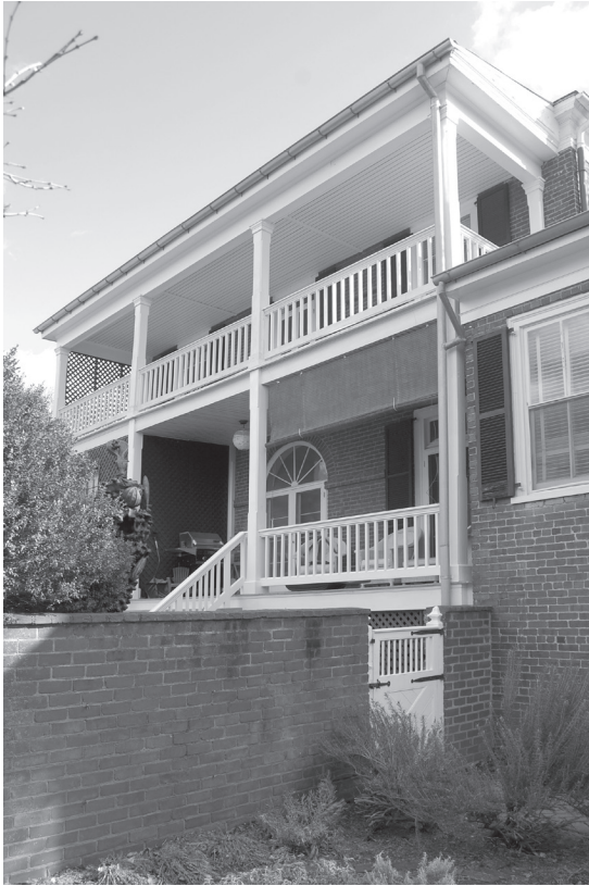
Pavilion IX from the southwest
