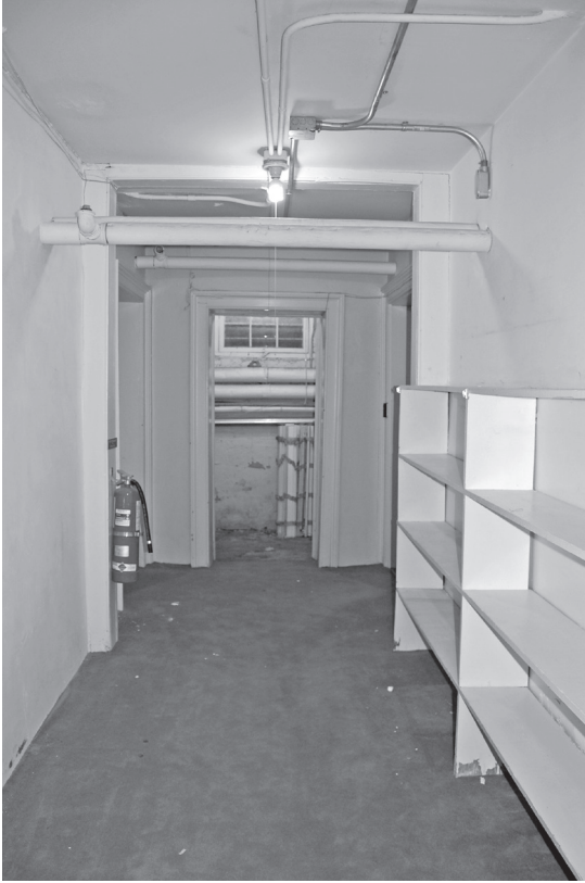
Room B02, looking east
