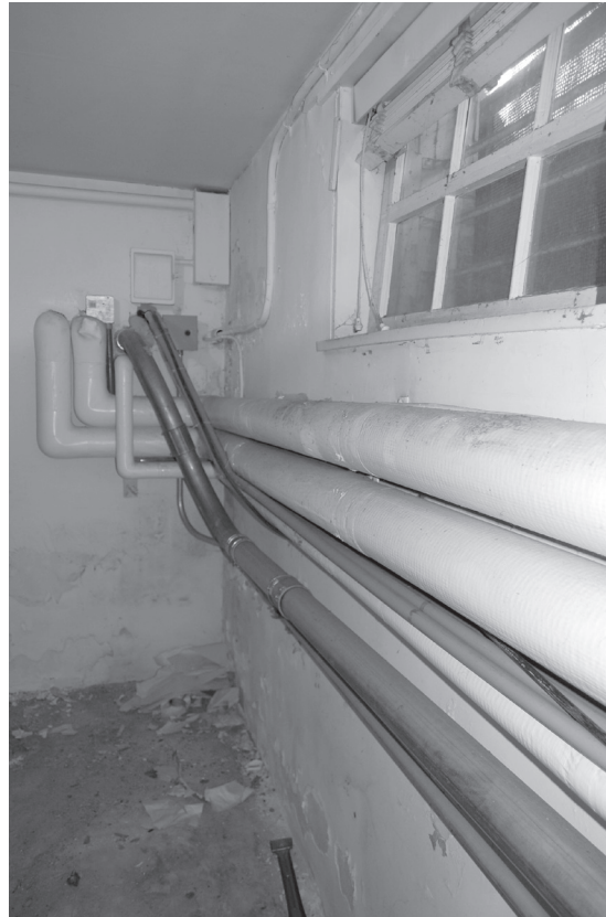
Room B05, looking north
