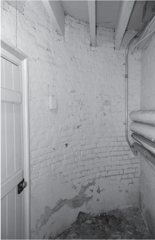
Room B04, looking north
