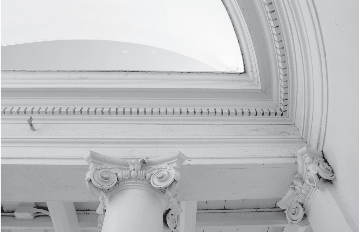
Column capitals and entablature of recessed east entrance
