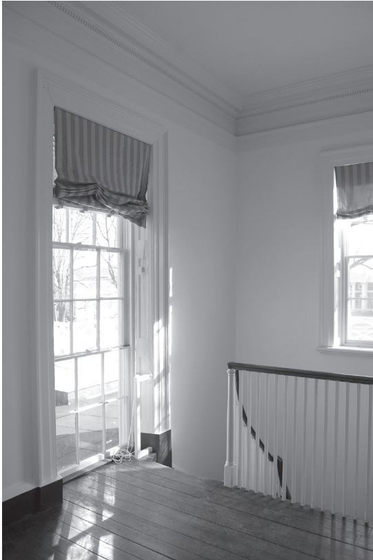
Room 201 (stair hall), looking southeast
