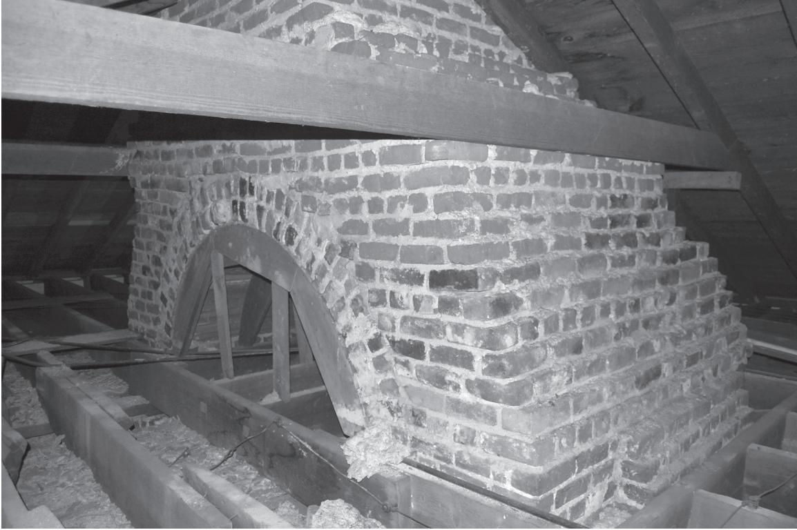
The chimney in the attic
