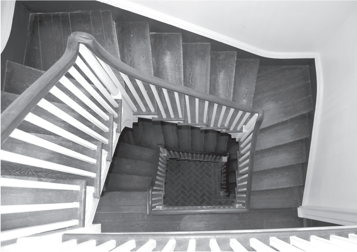
Room 104 (stair hall)
