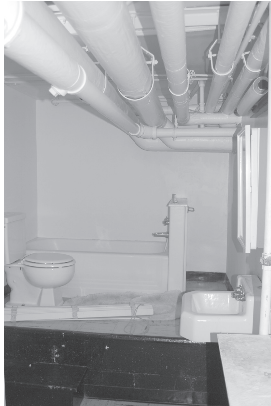
Room B09 (Bathroom), looking north
