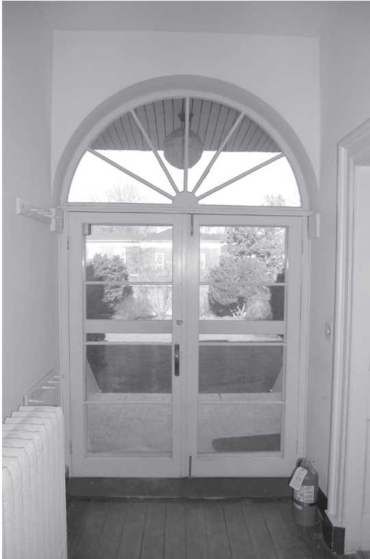
Room 105 (rear vestibule), looking west
