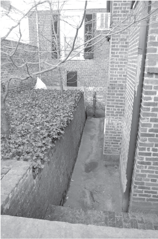
Light well and areaway along north elevation
