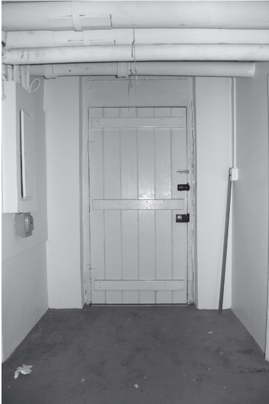
Room B08 (Vestibule), looking west
