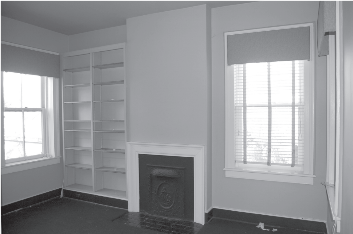
Room 108 (southwest addition), looking west
