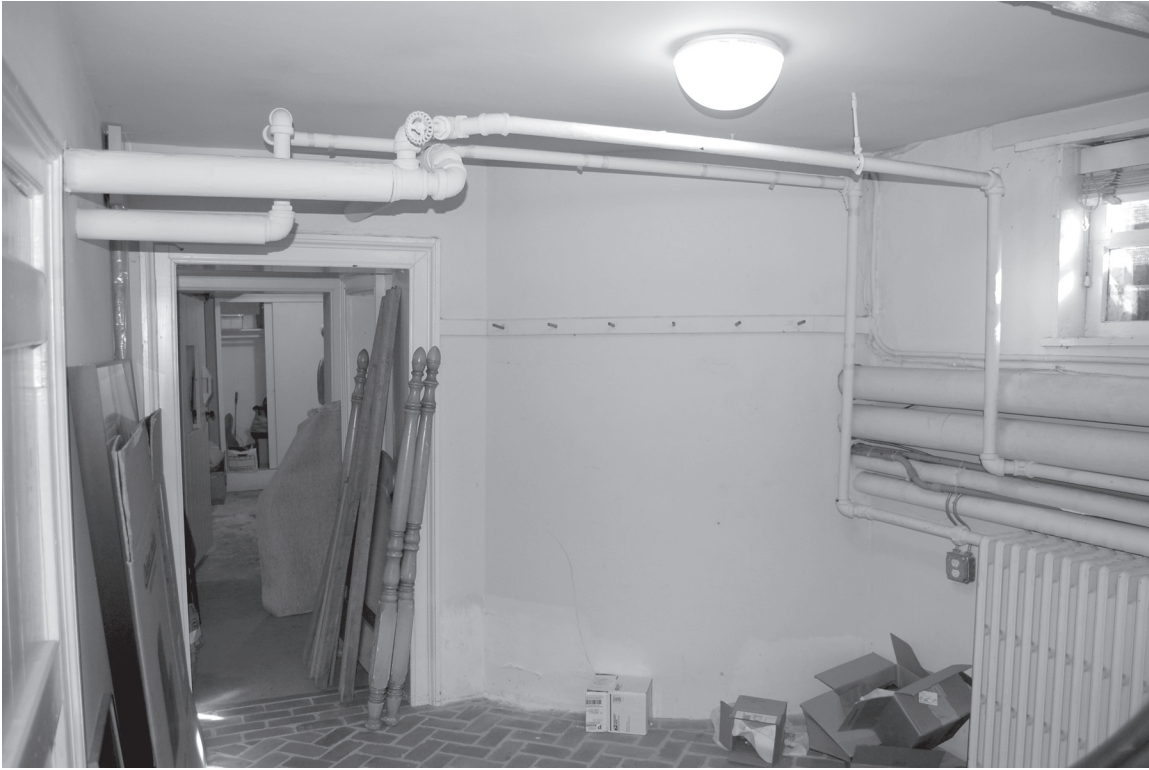
Room B01 (Stair Hall), looking north
