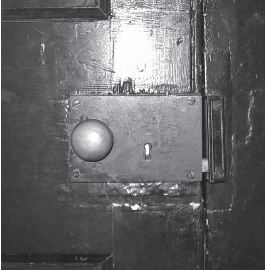
Rim lock on east entrance door (no. 1011)
