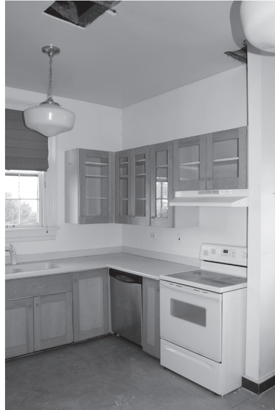
Room 106 (kitchen, looking northwest)
