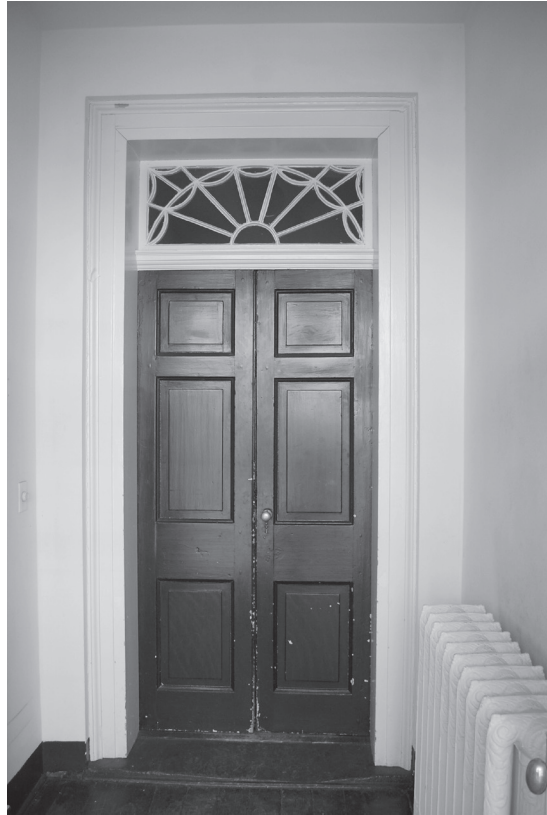
Room 105 (rear vestibule), looking east
