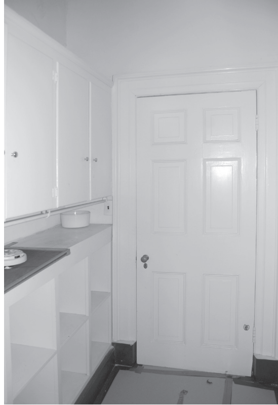
Room 207 (closet), looking southeast
