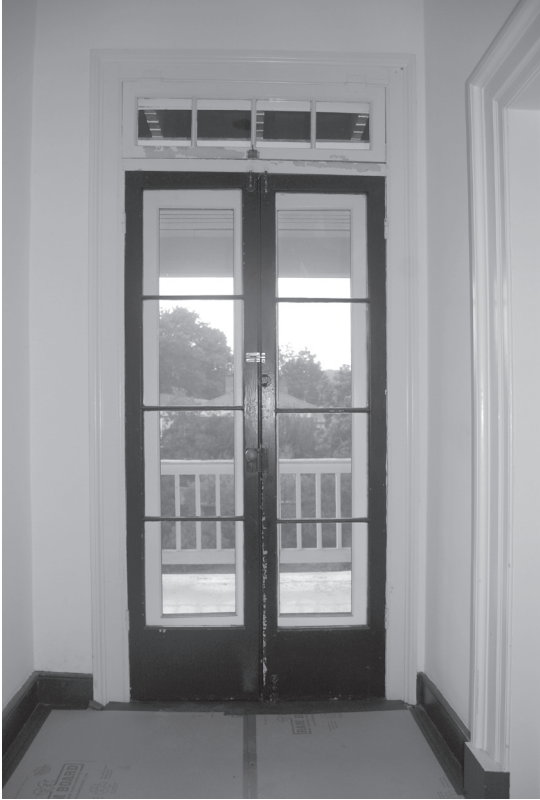
Room 206 (rear vestibule), looking west
