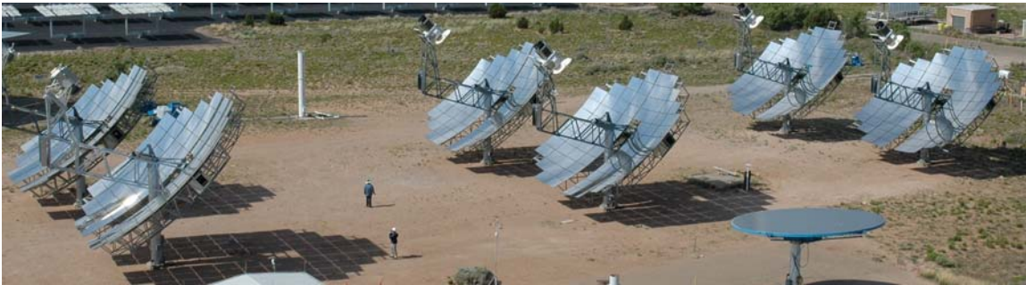
Figure C-3. Prototype 150 kW Dish/Stirling power plant at the NSTTF.
