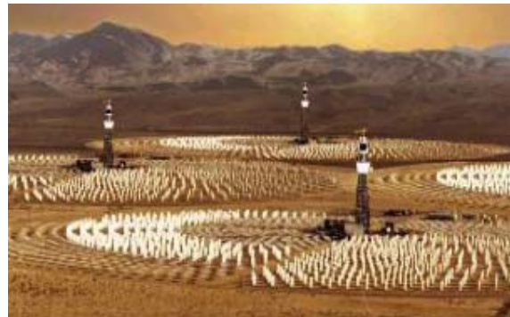
Figure 2.2-5. Advanced Power Towers
